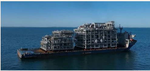
Arrival of Modules for Pluto Train Two - Dec 2024, Source: Woodside
