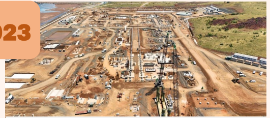
Perdaman Urea Plant Construction, Source: Clough
