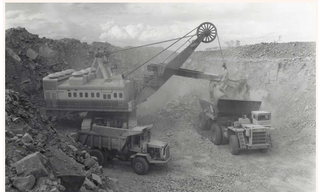
A giant power shovel and 95-ton trucks working on the Hamersley railway, May 1966 National Museum Australia
